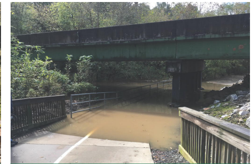
Greenway under Majors Road bridge during flood conditions.
