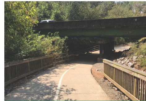
Greenway under Majors Road bridge during normal conditions.
